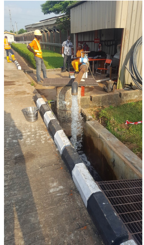
Test pumping a production well in Lagos, Nigeria.
