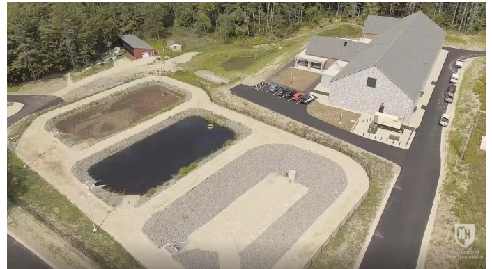
The new UNH/Durham Water Treatment Plant which went online in March 2020.
