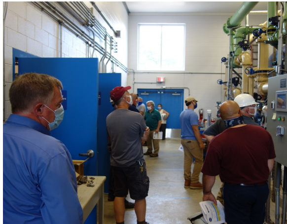
Construction Day in Merrimack 2020.
