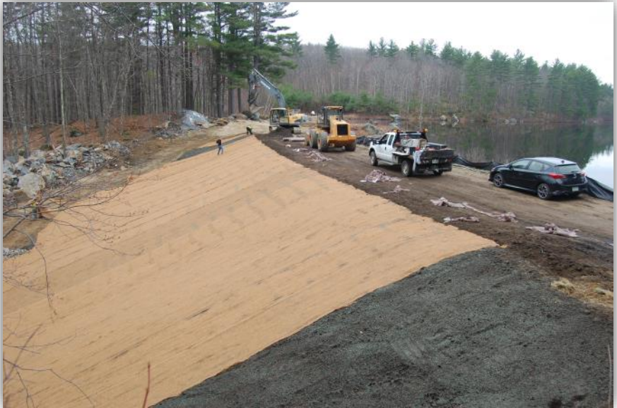
Dam repairs on the Rochester Reservoir.
