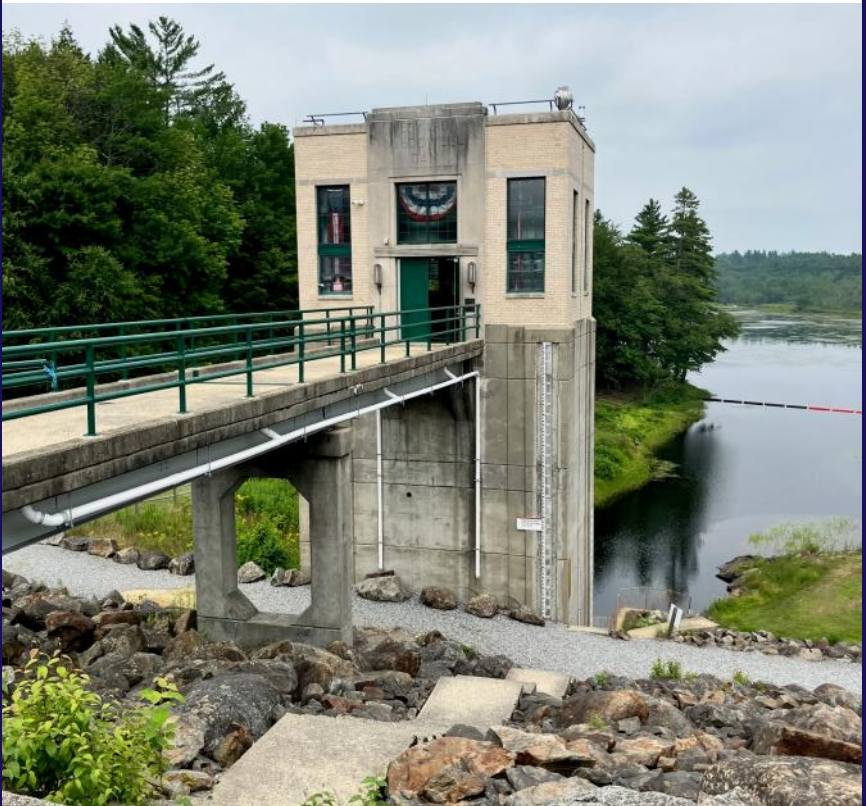
Edward MacDowell Dam, Peterborough, NH.
