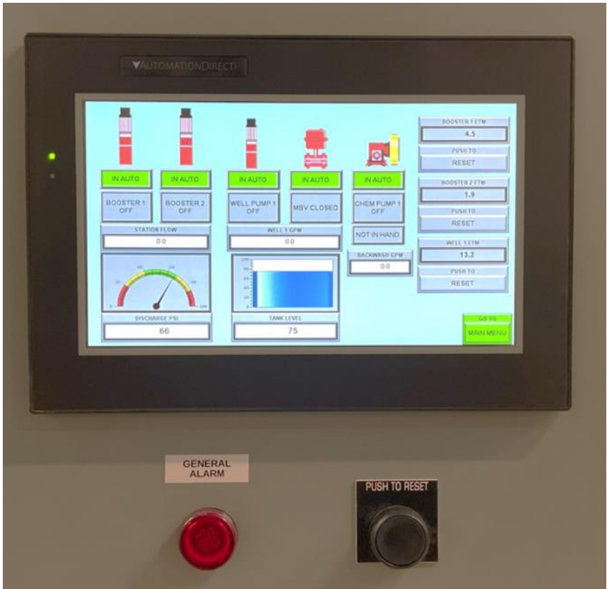
Automatic control panel. Operator Interface Unit (OIU) with touch screen showing the main screen
