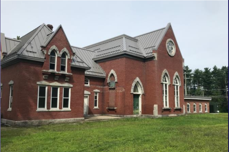
Manchester Water Works' Cohas Avenue pump station.
