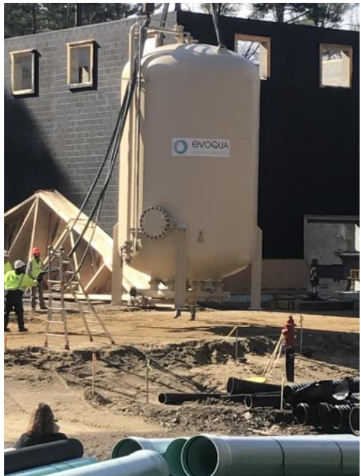
Installing carbon vessel at Wells 4&5.
