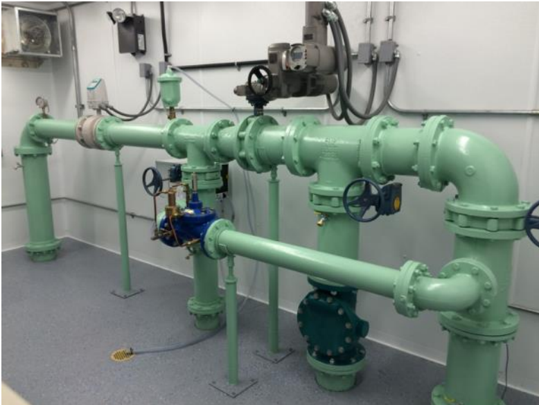
Figure 13 – Control Station Process Piping
