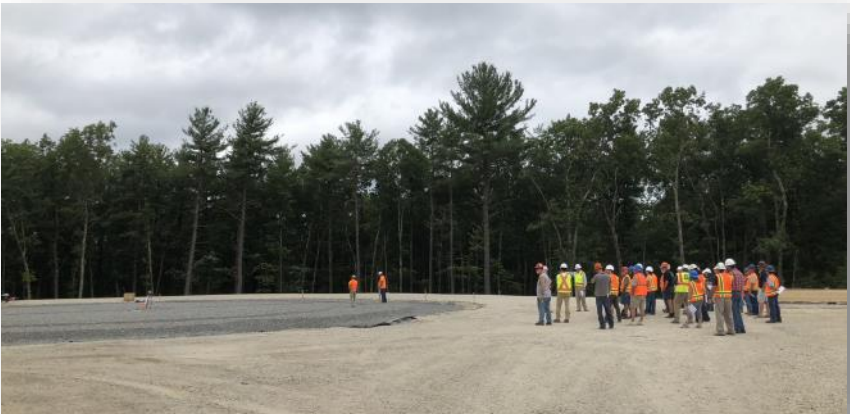
Site of Manchester Water Works' new 3MG tank in Londonderry.
