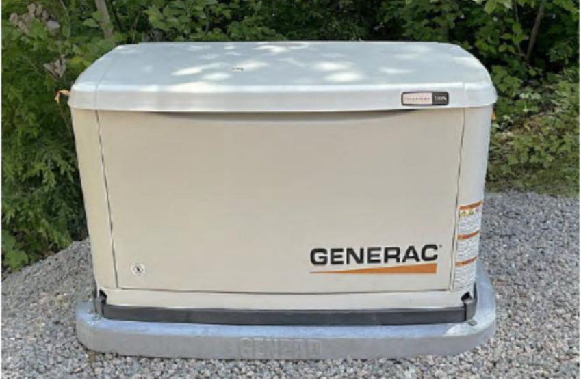
Generac Outdoor 24 KW, LPG, Standby, Automatic Genset for the Pump House
