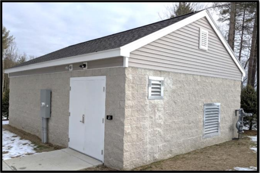
Bowman Place Booster Station (exterior).
