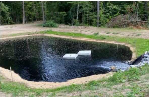
Figure 4-Initial Backwash of GAC at Startup- Well 4/5 WTP
