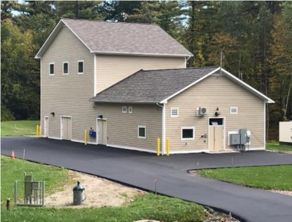
Figure 2- Completed Well #4 & #5 WTP
