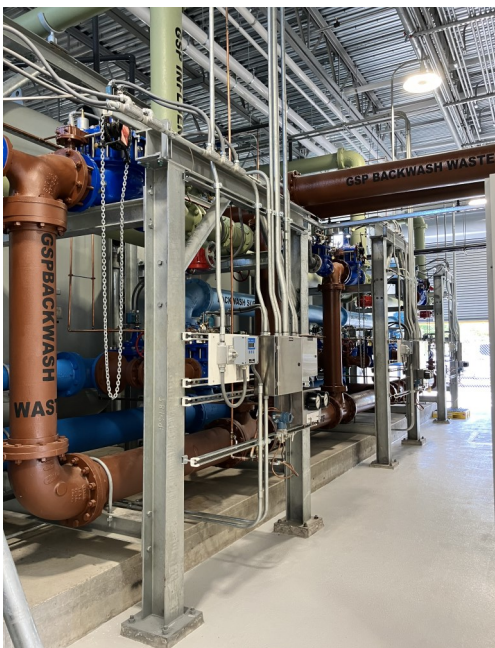
Inside Dover's Pudding Hill Treatment Plant, Construction Day 2024.
